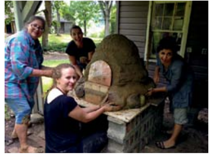
Mud Oven scavenged construction surplus locally dug clay bottles sawdust lots of people 2015
